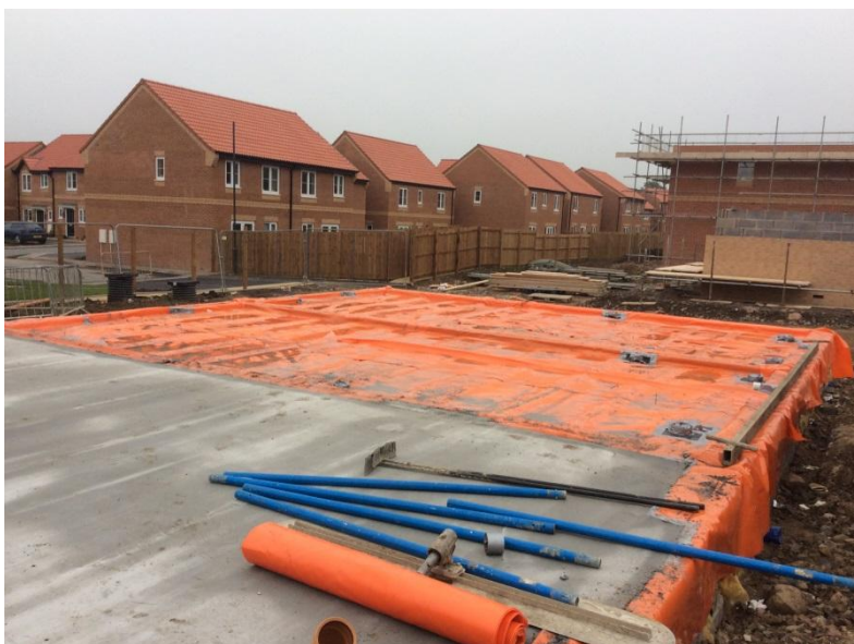
Figure 12 - membrane in place
