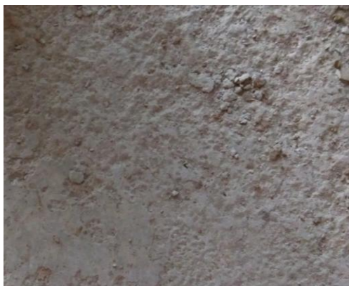
Figure 11 - frost damage
