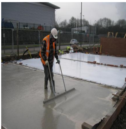
Figure 13 - dappling the SCC concrete
