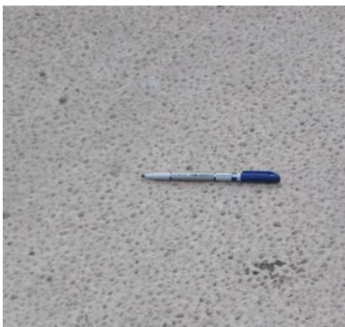
Figure 9 - rain damage
