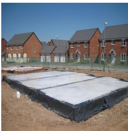
Figure 14 - curing agent applied
