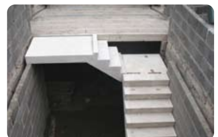
Precast Concrete Stairs
